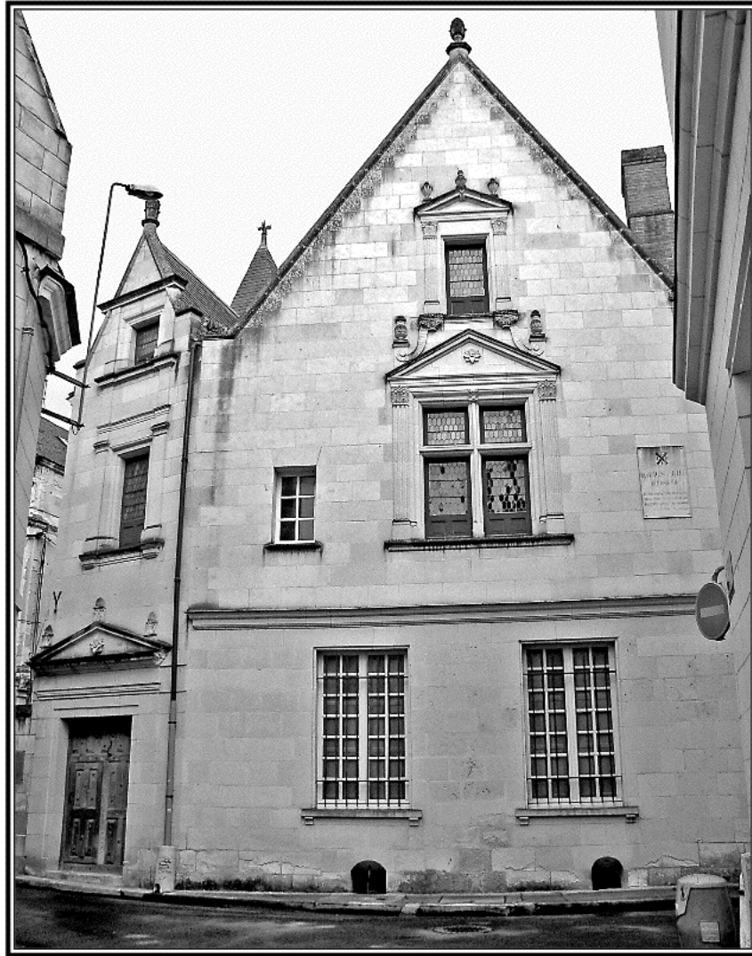
The Descartes family mansion in Châtellerault
